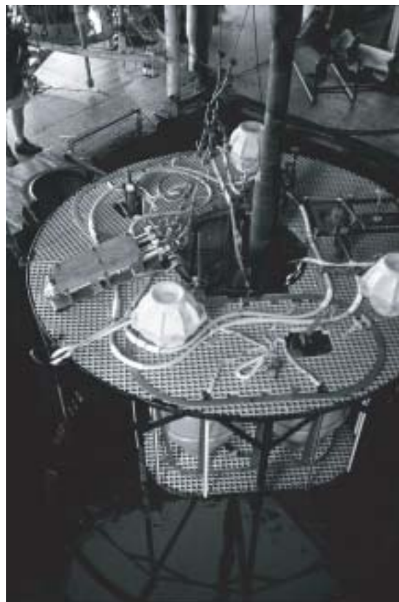
Figure 3 (right). Remotely operated vehicle (ROV) landing platform installed in Hole 1201D; lithium batteries for ION seismometer are on lower level.
