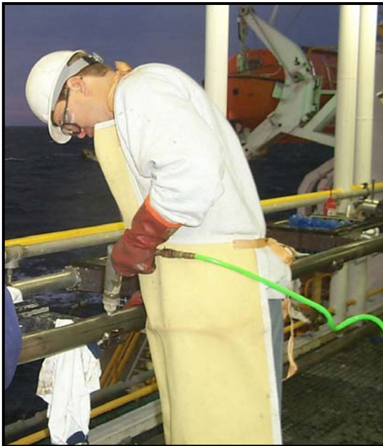
Figure 18. Drilling holes in liner.
